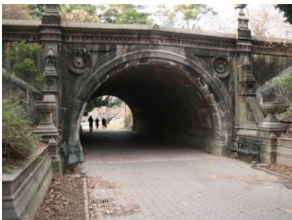
Pont Cleft Ridge Span
